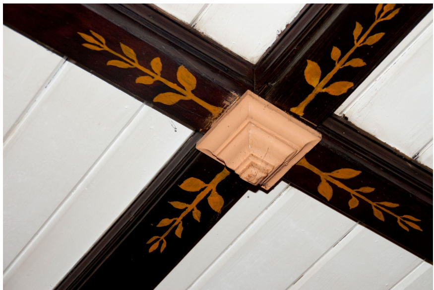
Interior ceiling beam
